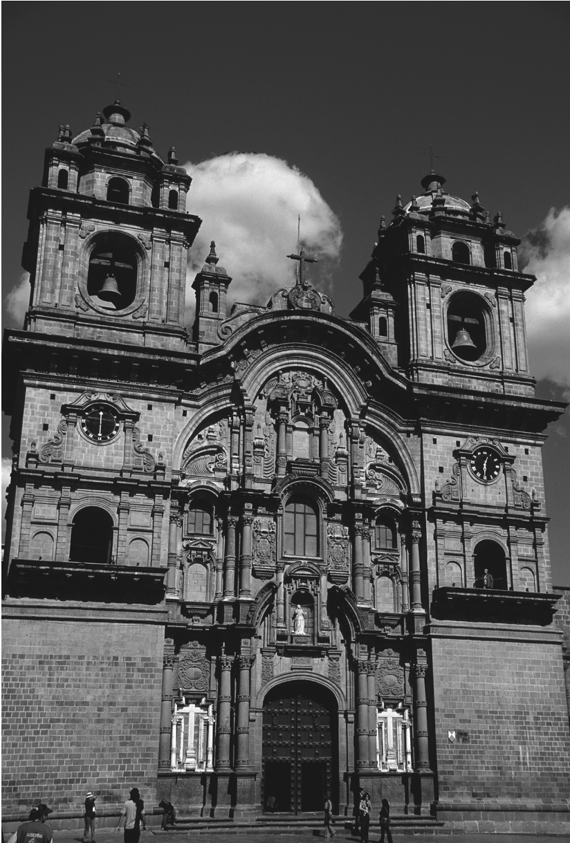
Figure 13.1. Church of the Transfiguration, or Compañía, Cuzco. Façade. Photo by Gauvin Alexander Bailey.
